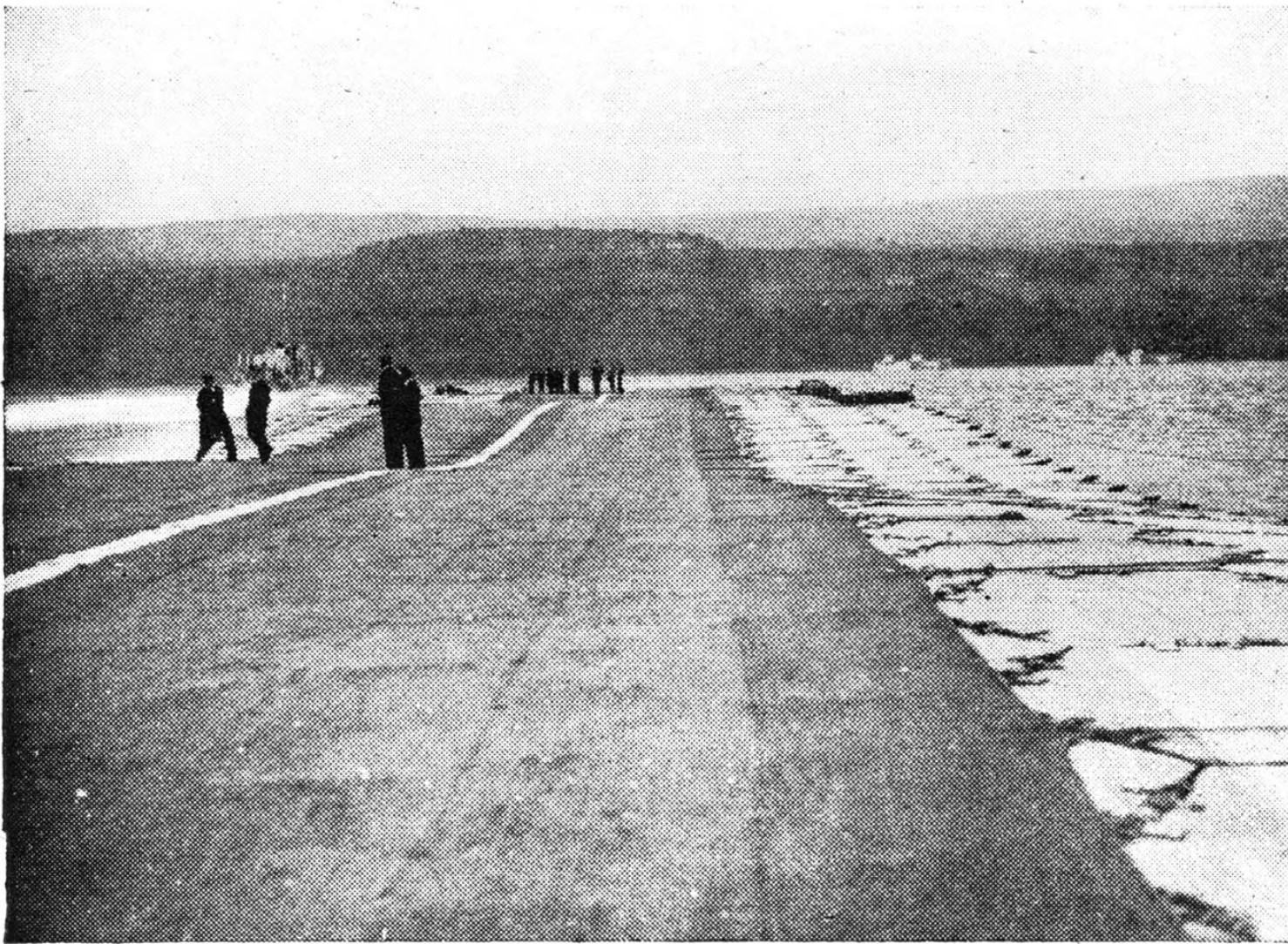
"LILY": The Navy's experimental floating airstrip measuring 520ft. x 60ft. is here seen undulating in the wash of a passing launch. A 9,000lb. aircraft has successfully used it.
