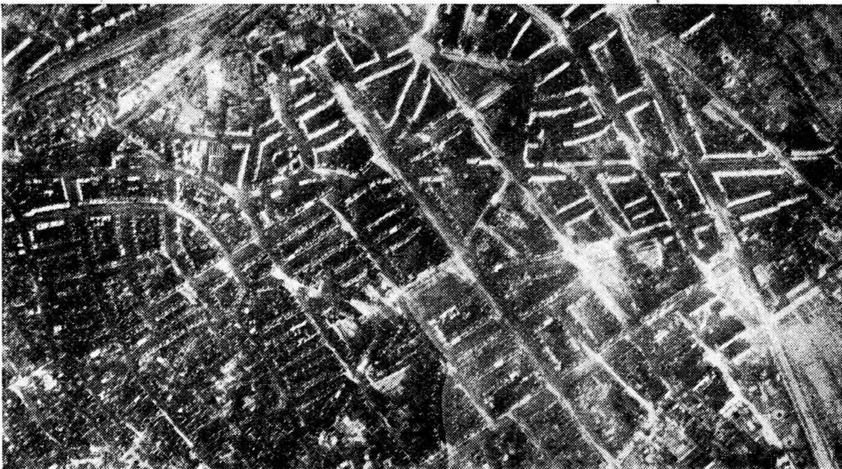
THE AFTERMATH.—The same portion of Hanover photographed after the raid. Very few roofs remain or buildings intact. The whole area was devastated by fire.
