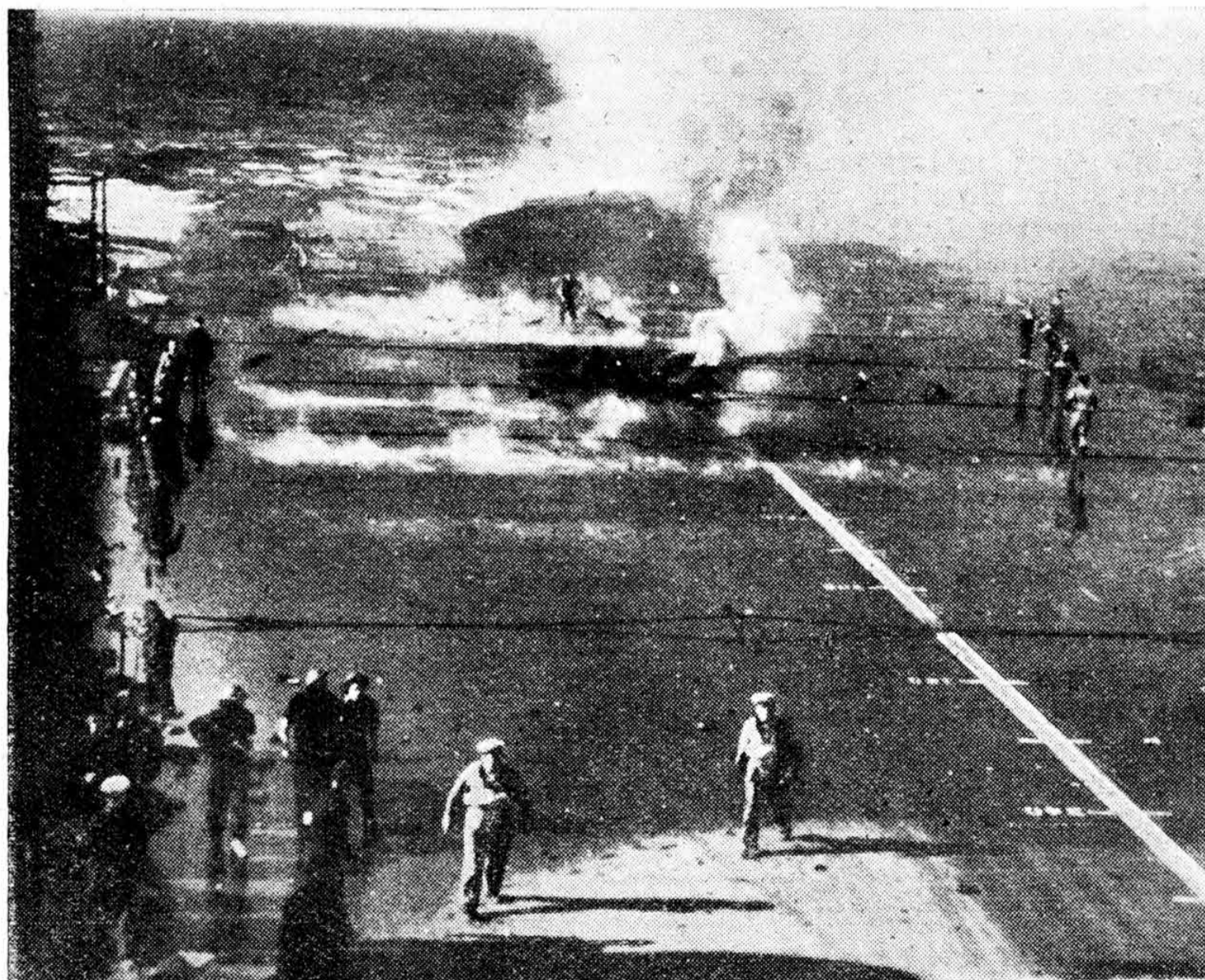
DIRECT HIT. —Part of the flight deck of the aircraft carrier Illustrious after a direct hit from a bomb on January 10, 1941. Stores, stowed in the roof of the hangar just below, caught fire and smoke can be seen coming through the bomb hole. The deck was so hot that water poured on to it turned to steam. The after lift was raised bodily from its place and can be seen beyond the hole. The carrier reached Malta and later crossed the Atlantic to America for repair.
