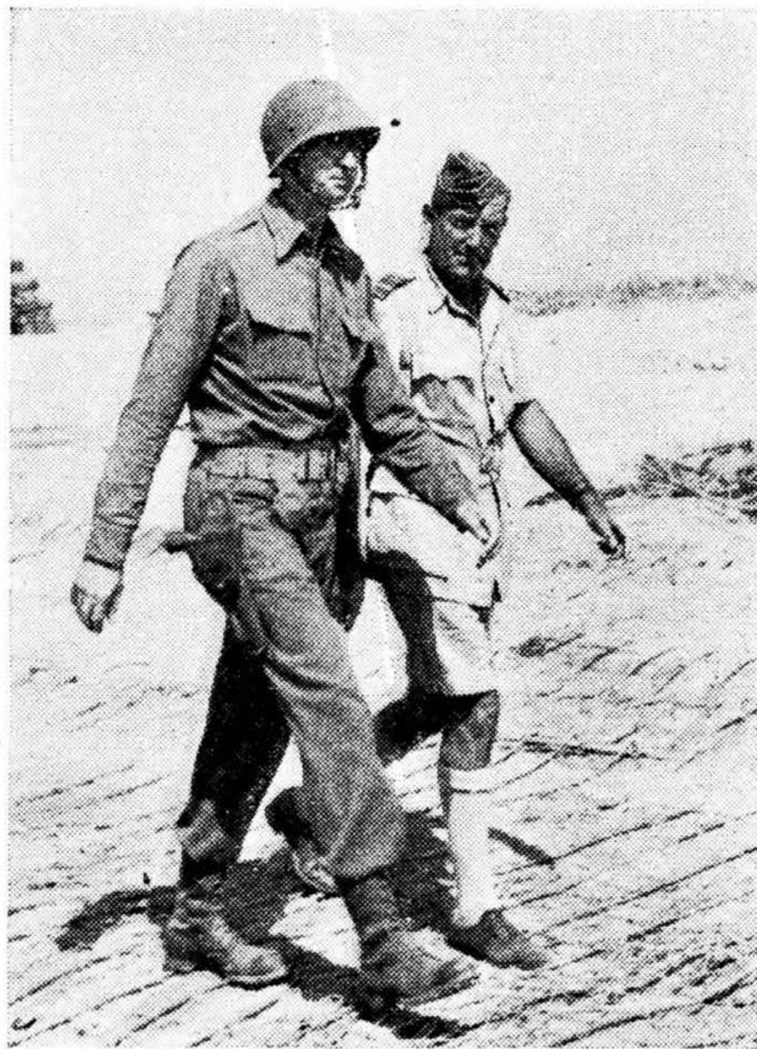
STEEL ROAD. —General Mark Clark, G.O.C. Fifth Army, with Air Marshal Sir Arthur Coningham on a beach road near Salerno. The surface is of steel rods and wire to carry heavy transport over soft sand.
