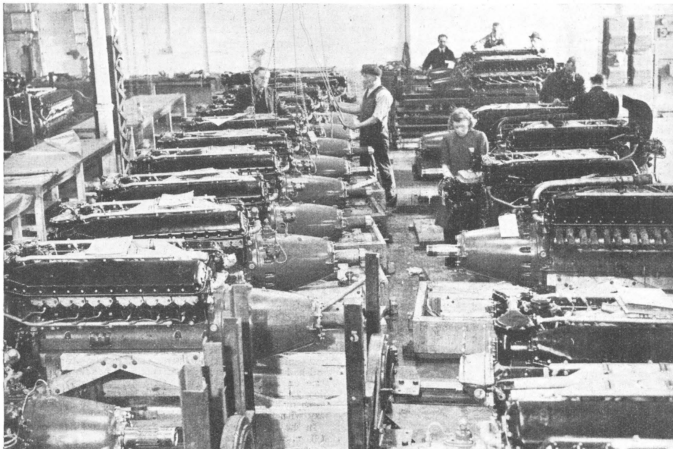
ALLISON IN-LINE.—Allison V-1710-C15 motors ready for the test bed after overhaul at a Maintenance and Repair Depot somewhere in England. On each motor may be seen its own log-book.
