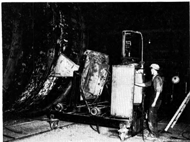
FIG. 7 PORTABLE X-RAY APPARATUS USED IN FABRICATING PLANT
