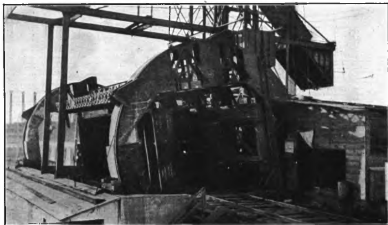
FIG. 2 VIEW OF ROTARY CAR DUMPER
