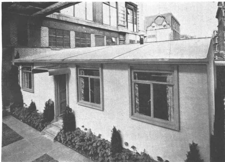
VIEW of the aluminium house illustrated above shows the light-metal roof. Below is seen the lounge, looking towards the fireplace.
