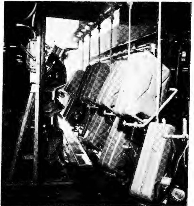
Fig. 2. Large 504 kW Infra-Red Plant.
