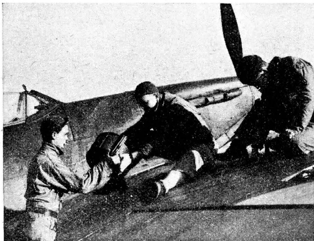
BIGGER STUFF. —A drum of shells for one of the two 20-mm. cannon in the same Spitfire VB. The cannon are loaded from above, the machine-guns from below.
