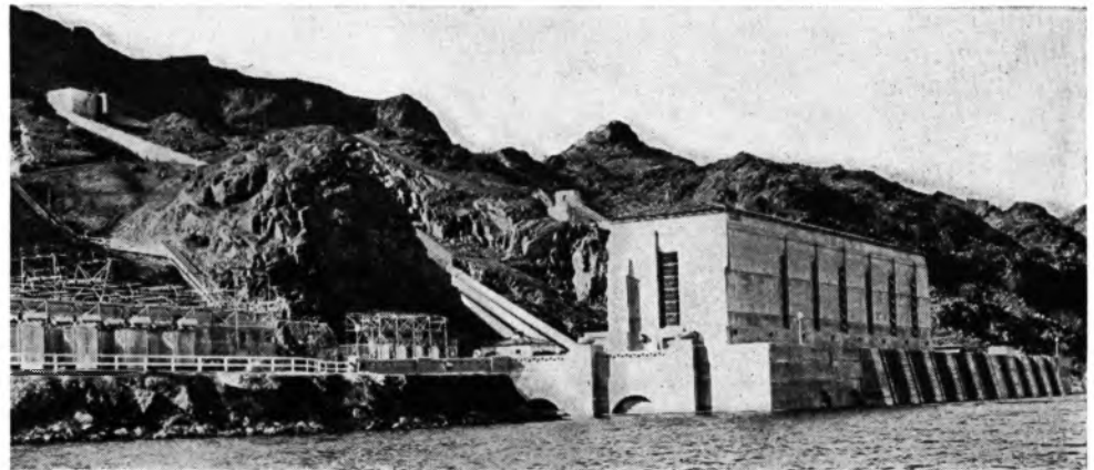
FIG. 3 THE INTAKE PUMPING PLANT ON THE COLORADO RIVER
