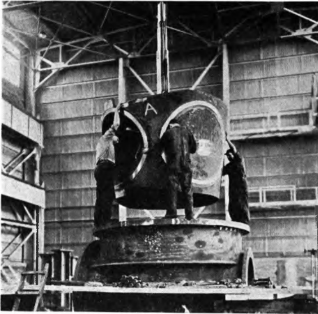
FIG. 5 ASSEMBLING THE BODY AND PLUG OF A 42-IN. BY 58 3 / 4 -IN. TAPERED ROTOVALVE; S. MORGAN SMITH COMPANY
